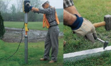
A minimum 30" piece of Die cut knockout is punched out of post at desired location. 12 gauge Telespar square steel tubing one size larger than the intended signpost
